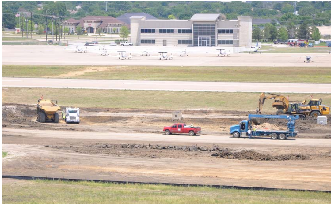
West Parallel Taxiway Construction
